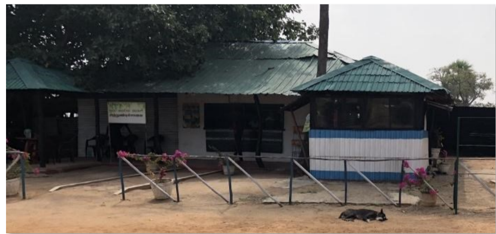
Sittrundisaalai A34 , Junction of Mankulam-Mullaitvu Road and Puthukudiyiruppu-Mulliyawalai Road, Mullaitivu
